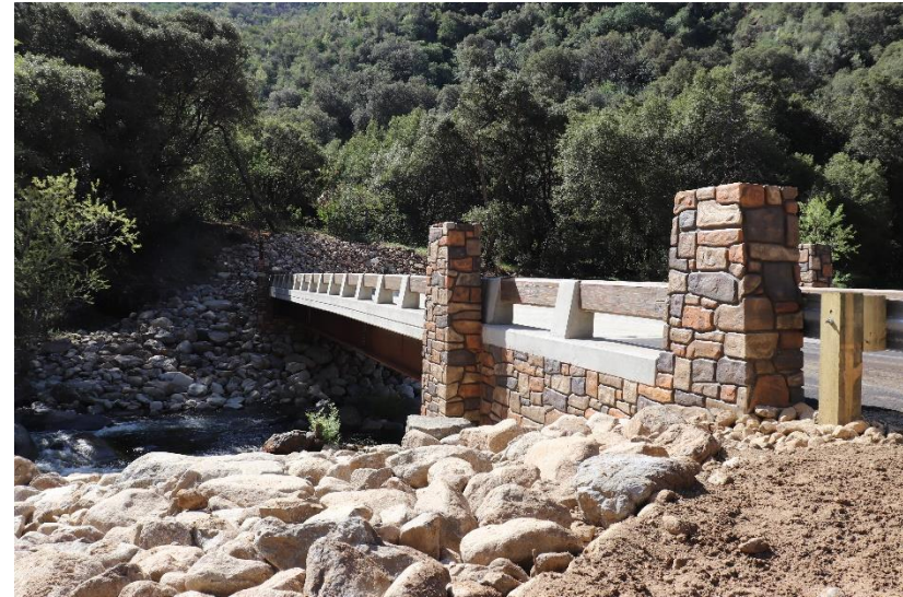
Mineral King Road over S. Fork Kaweah River Bridge (Three Rivers, CA)
